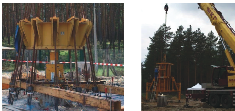
Figure 3: Static load test (left) and dynamic load test (right)
