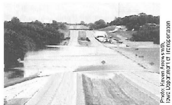
Figure 1: Bridge-submerged flow in Iowa in 2008
