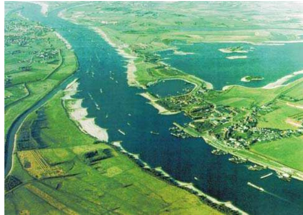
FIGURE 3. AREAL VIEW OF GOYNES AT THE WAAL RIVER
