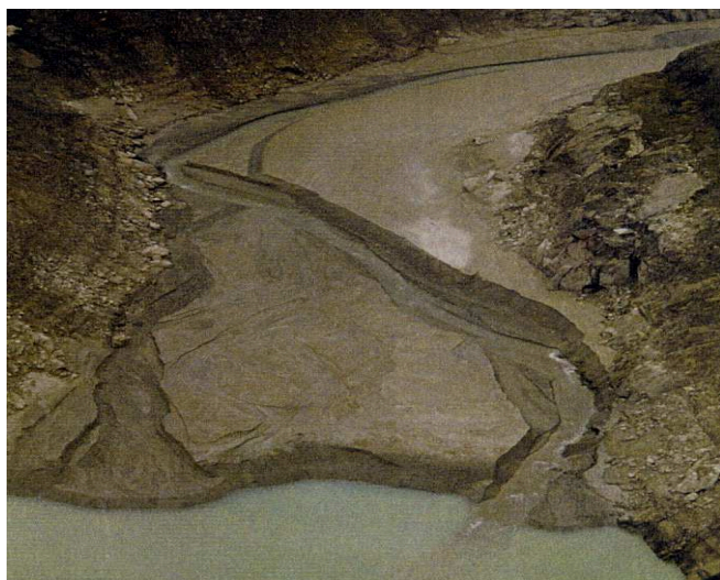
Figure 2. Flushing channel in reservoir upstream of Gebidem dam during drawdown operation
