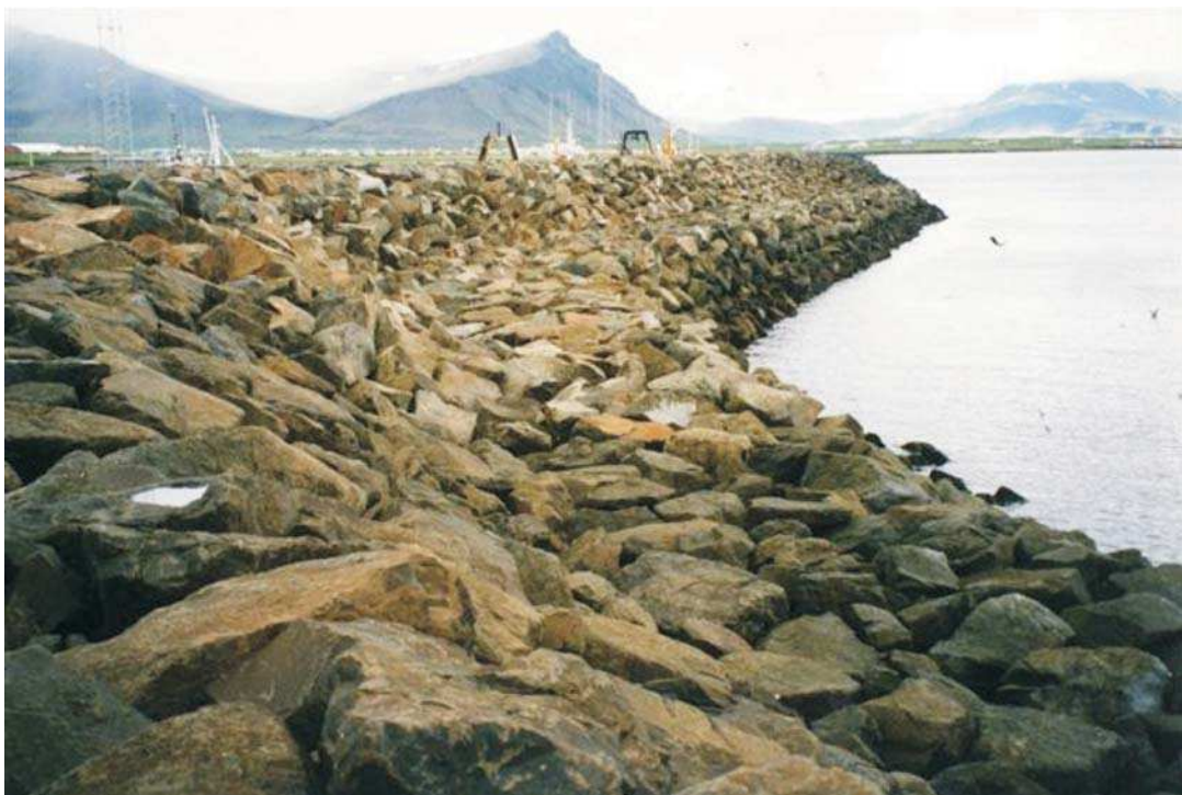
Fig. 6.7: Icelandic Berm breakwater
