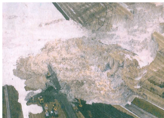
(b) Bernburg tailings dam, Germany (2007) (Ballard, 2008 and Vanden Berghe, 2009).
