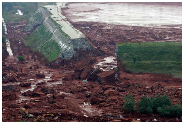
Kolontárt Devecseri tailings dam, Hungary (2010)
