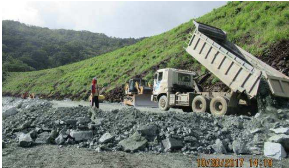
Figure 6: Placement of stabilizing fill at the Main Dam
