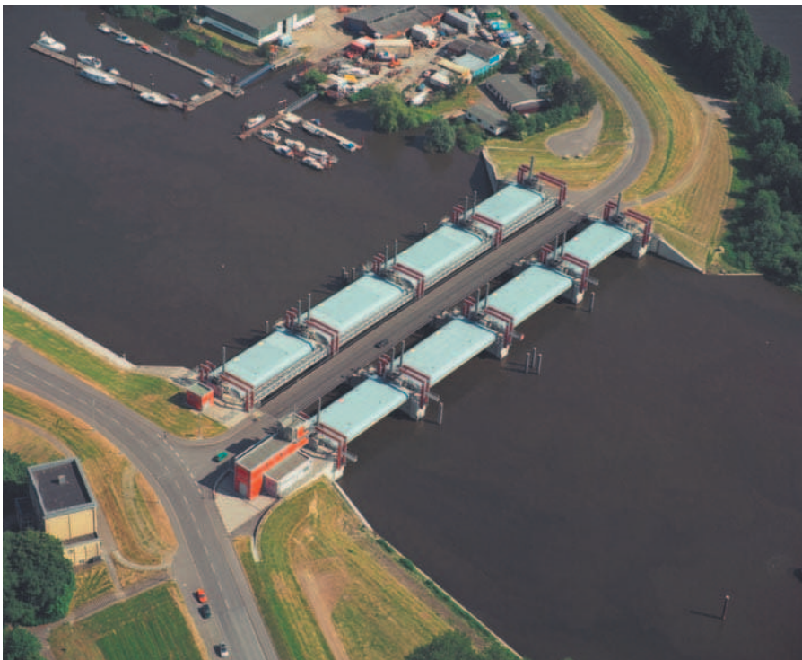
Fig. 12: Aerial photograph of the Billwerder Bucht Barrier/© HPA Hamburg
