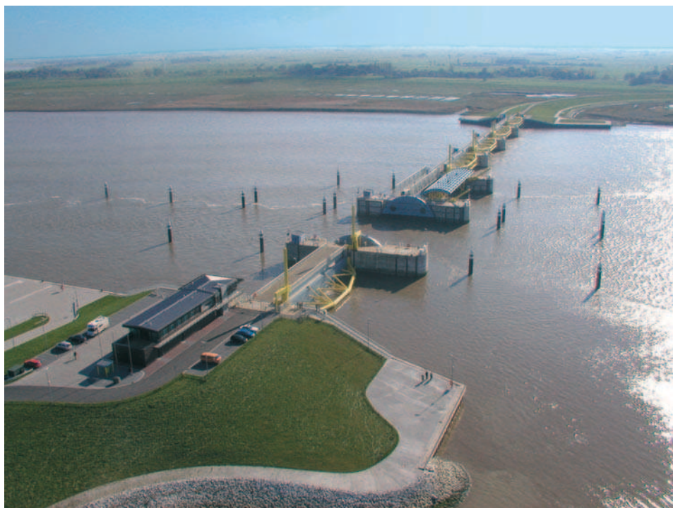
Fig. 2: Aerial photograph of the Ems Barrier/© NLWKN Aurich
