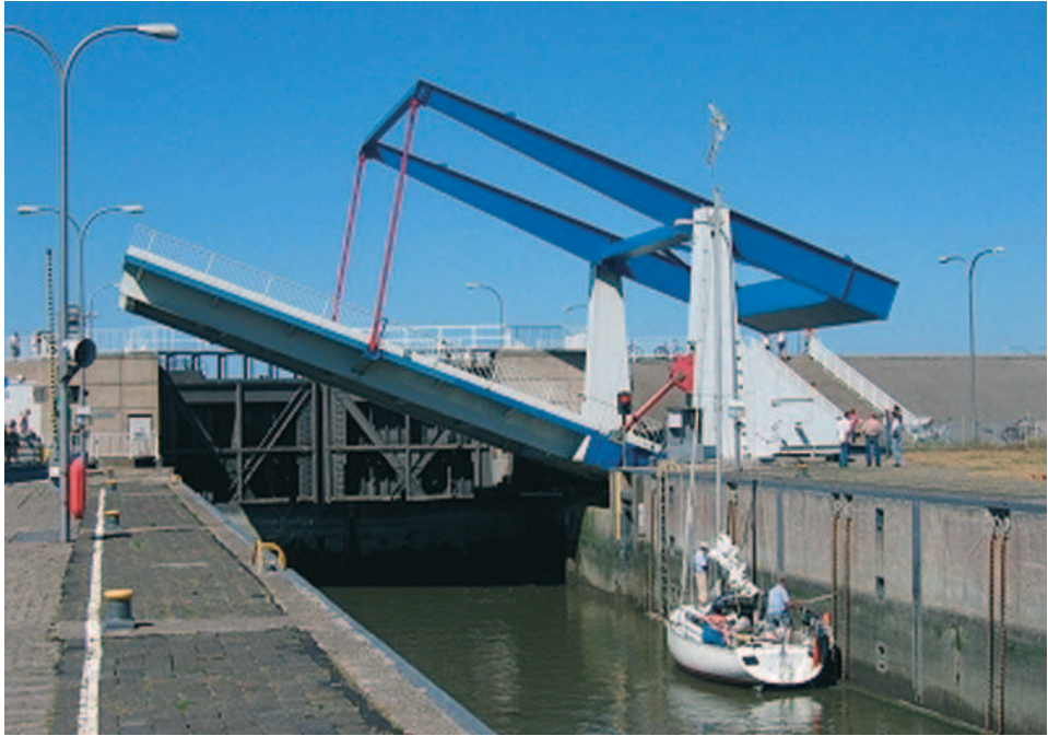
Fig. 7: Lock chamber with bascule bridge/© WSA Tönning
