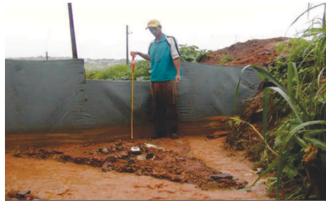
Figure 4.4. Upstream view of sediments retained by the fence.
