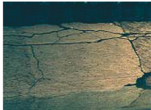
Figure 9.5. View of an old concrete lining (Poulain & al., 2000).
