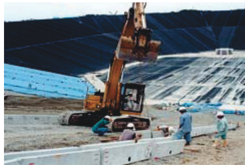
Figure 9.4. Construction of sheet connection structure (Takimoto & al., 2002).
