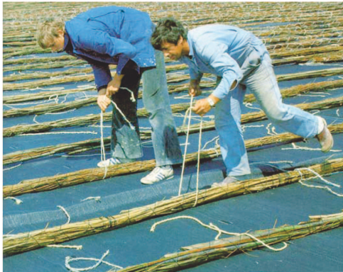
Figure 4.5. Preparing a fascine mattress (willow mat).
