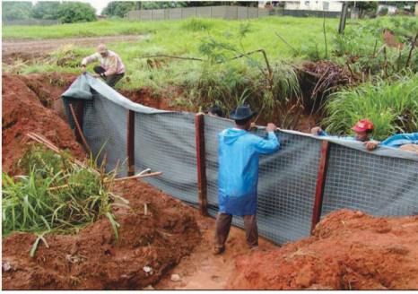
Figure 4.3. Downstream view of the silt fence construction.
