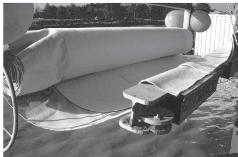
Figure 9.6. Staggered GCL and sandmat to be unrolled under water.
