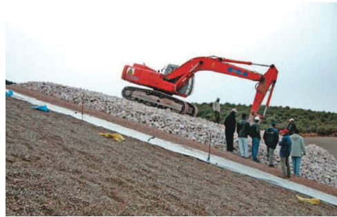
Figure 9.3. On slope GLS testing for Afouer pond (Fayoux & al., 2005).
