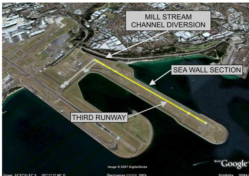
Figure 1. The runways of Sydney's Kingsford Smith International Airport with Millstream Diversion and Seawall.
