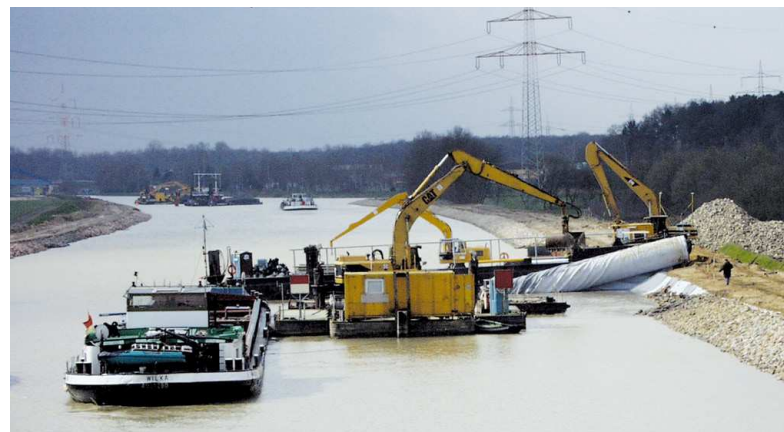
Fig. 2: Installing a geotextile on a federal waterway
