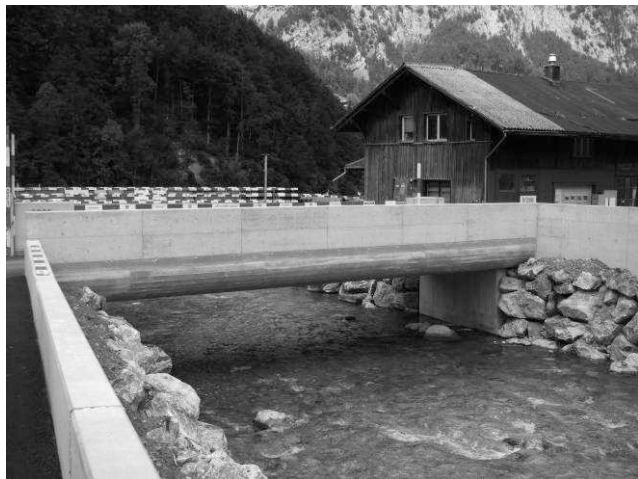
Figure 9. New baffle bridge at River Chirel, Switzerland
