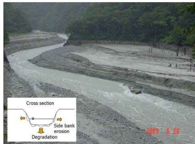
Photo 1 Sediment Flushing in Dashidaira Reservoir
