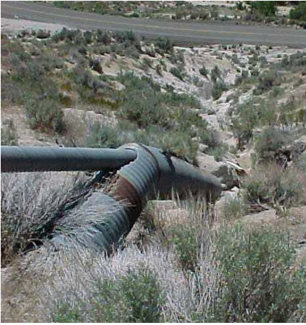
Figure 1. Culvert with free discharge at top of slope
