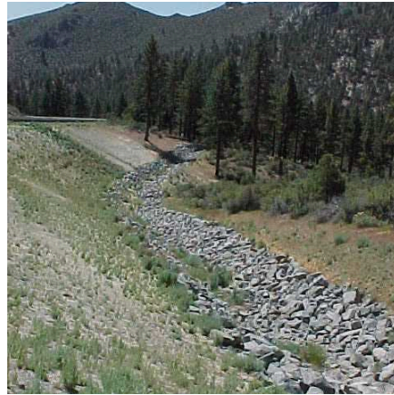
Figure 4. Channel lined with rip rap
