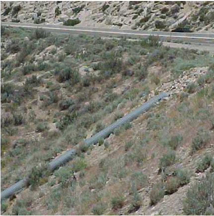
Figure 3. Culvert with a pipe slope drain
