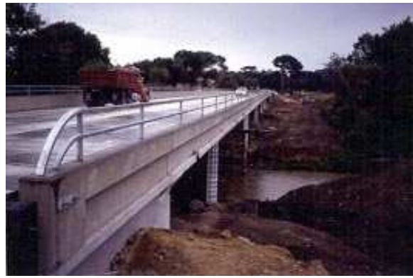
Figure 8: New Highway 1 Bridge with Pier Wall Construction under way (photo by Author, 1995)
