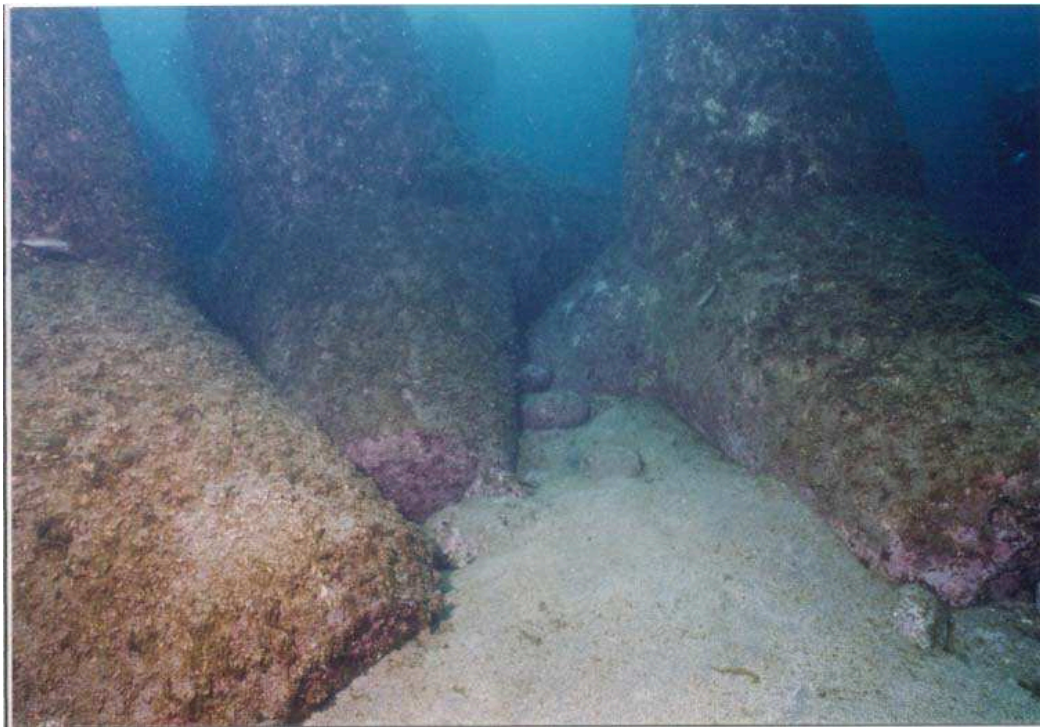
Fig. 2 - Video-captured scour hole
