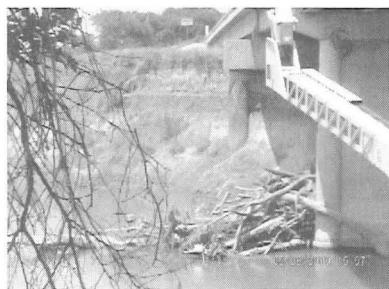
Figure 7. Exposed drill shaft
