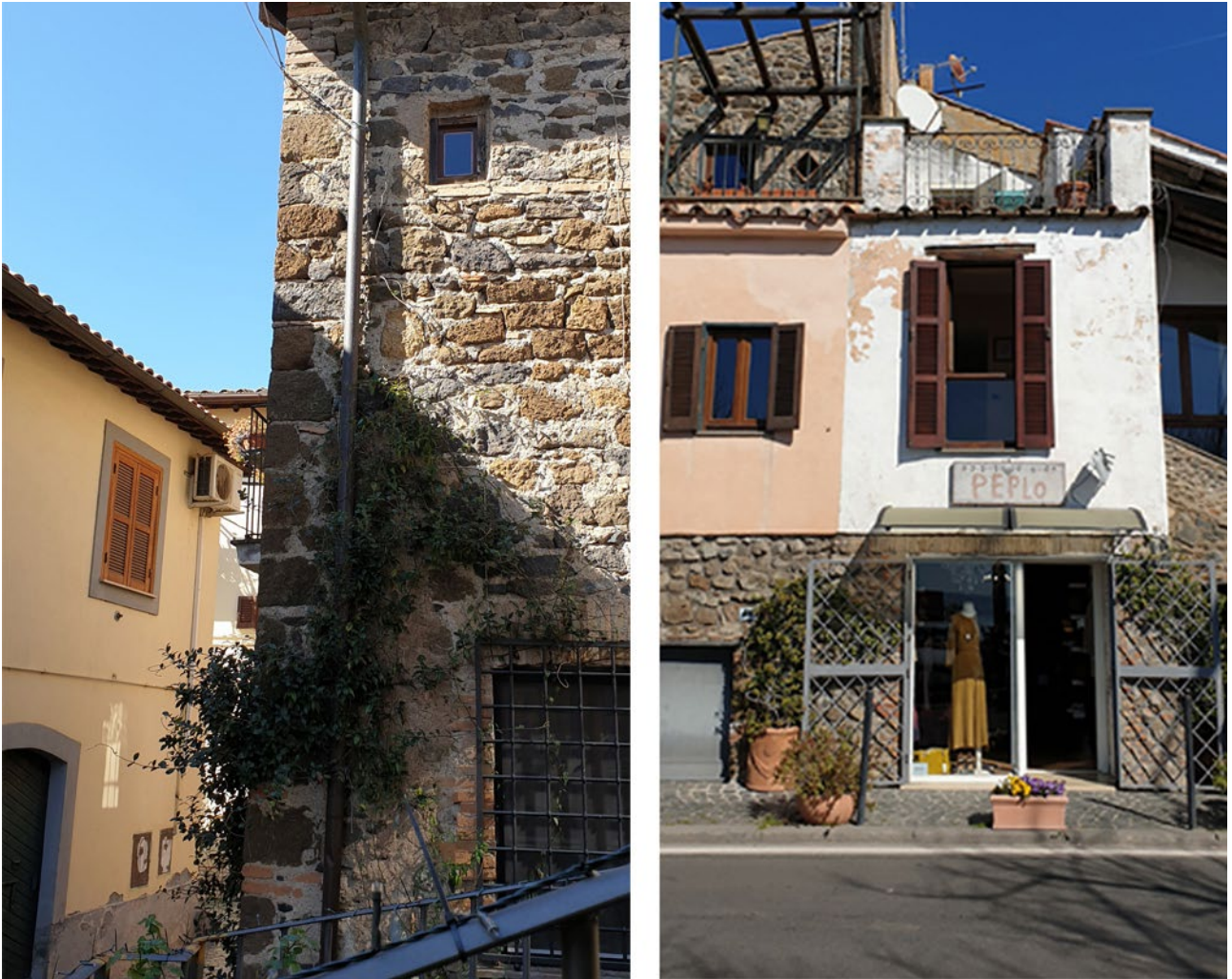
Figure 5: Historical centre, wooden windows fixtures. Source: photos by authors.
