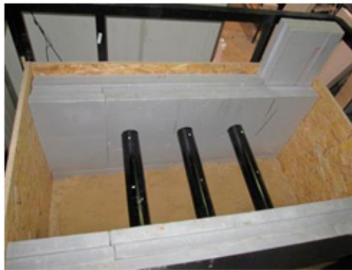
Figure 2. Placement of power cables in the sand.
