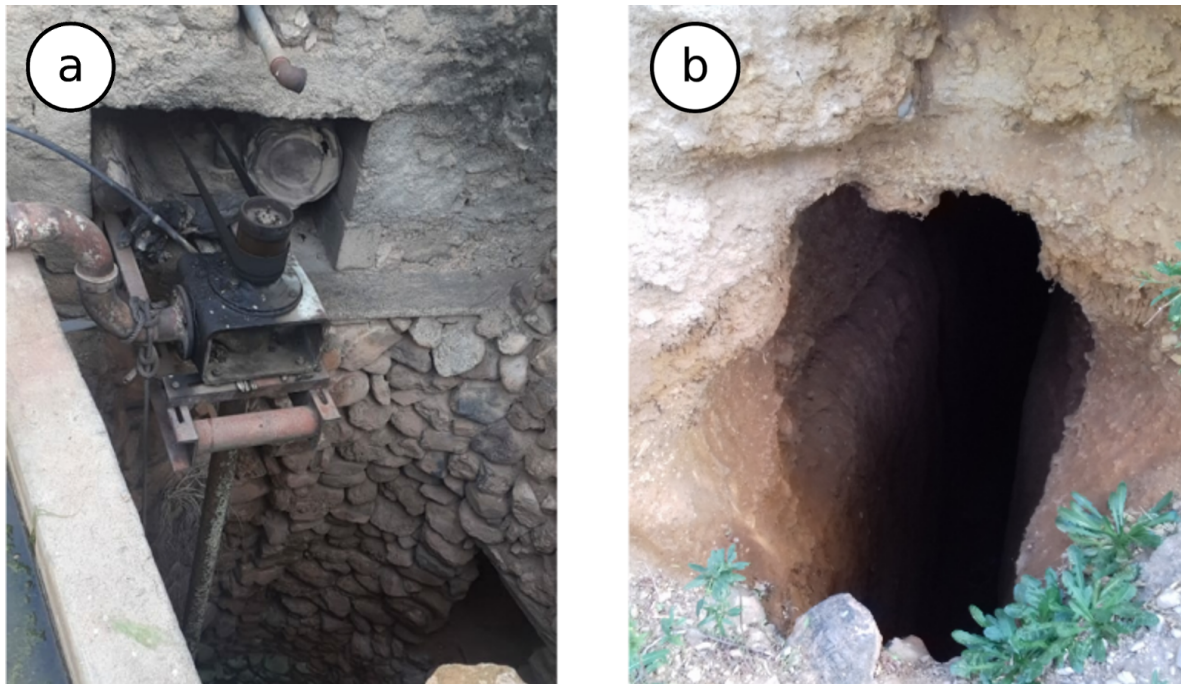
Figure A1. Wells for irrigation adopted in Assaragh: (a) modern with mechanical pump, (b) and traditional.
