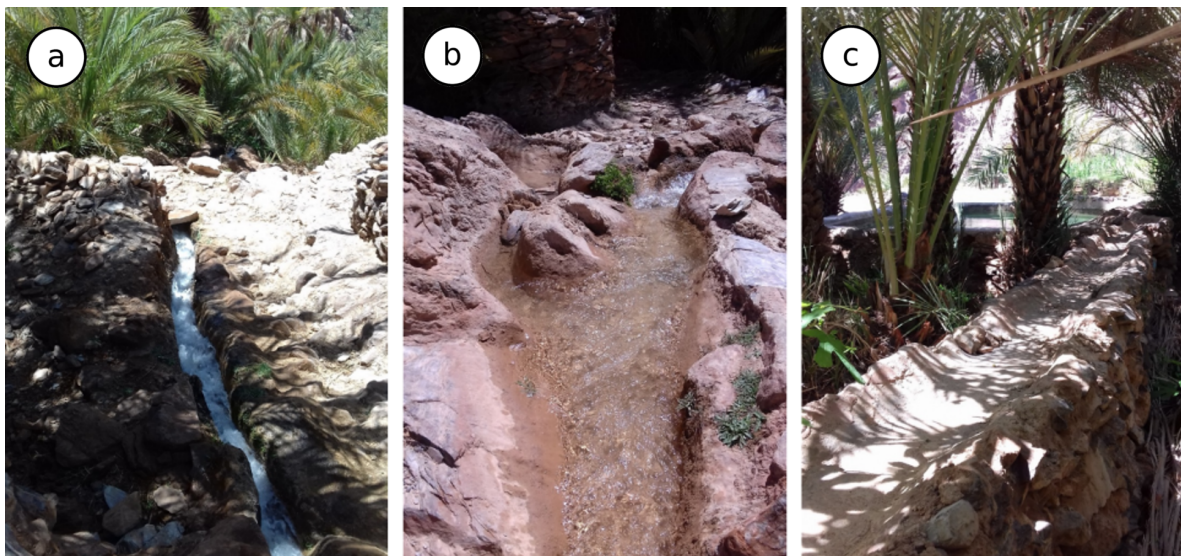
Figure A2. Traditional channels for water irrigation; the walls of the channels are covered by calcium carbonate natural deposits, due to the water filtration through the limestone in the basin. (a) A steep channel. (b) Bifurcation and repartition of the flow. (c) A horizontal channel built and naturally calcified on a dry stone wall.
