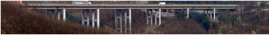
Fig. 3. Lateral view of the Rio Torto viaduct.
