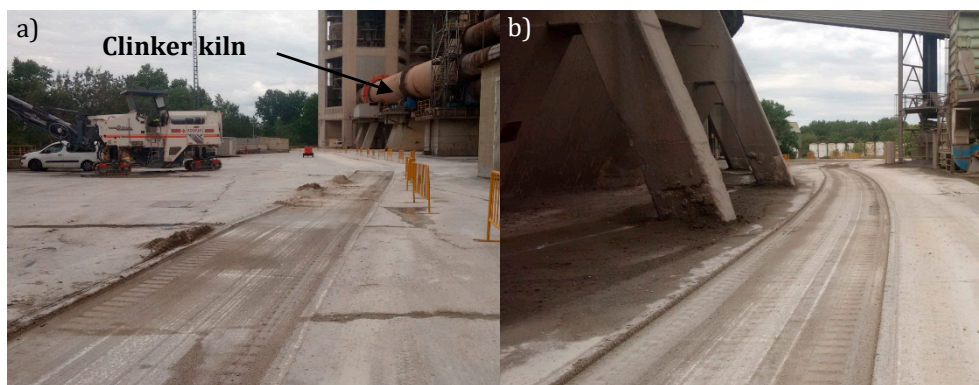
Figure 8. Original concrete pavement (a). The appearance of the cold-milled box (b).
