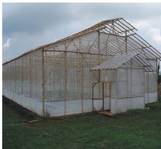
Gambar 1. Rumah plastik bambu ( Bamboo plastichouse )
