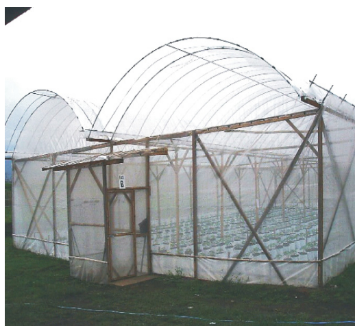
Gambar 2. Rumah plastik kayu-metal ( Wood-metal type plastic house )
