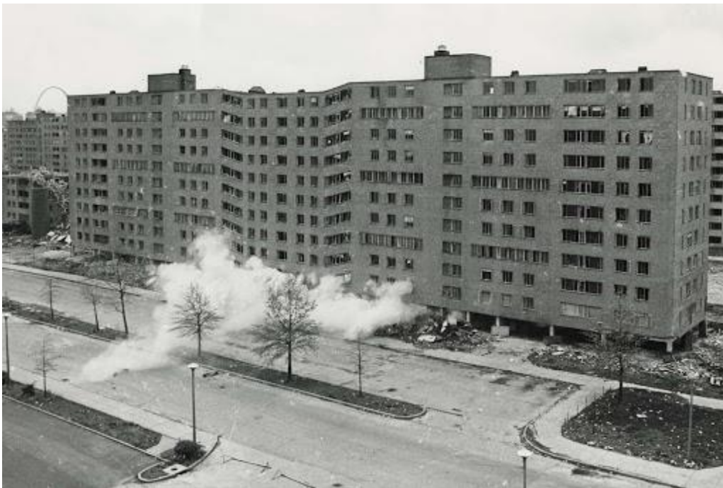
Figure 2: Pruitt-Igoe Housing Projects Demolition, Chicago, Illinois
