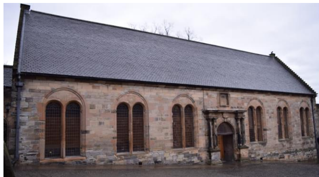
Figure 7: South façade of the Chapel Royal in Stirling Castle.
