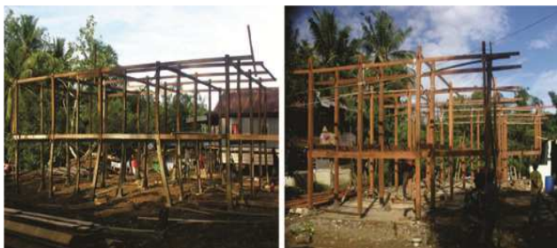
Fig. 3. Comparison between old and new Bugis building structure
