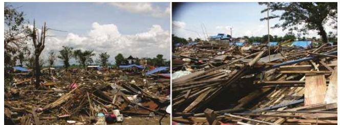
Fig. 11 Total damage due to tornado
