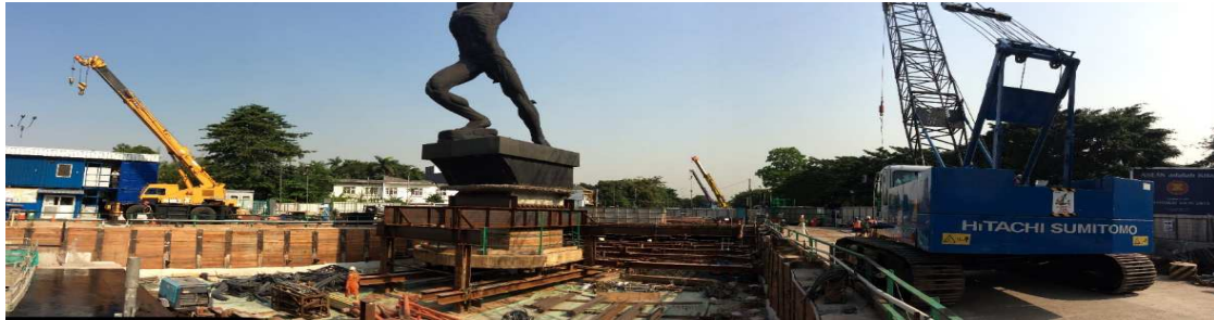
Fig. 10 Challenge in excavation under the statue at Sisingamangaraja
