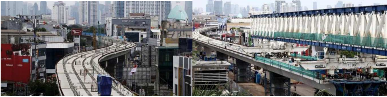
Fig. 7 The challenge of Traffic Diversion for Construction in the South Corridor
