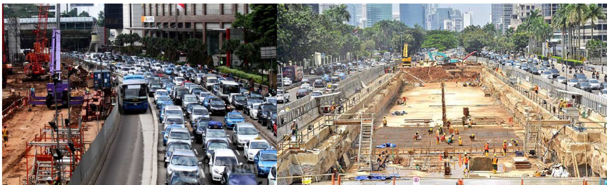
Fig. 8 Managing the traffic flow around the excavation in the North Corridor
