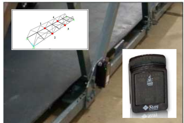
Fig. 3 Accelerometer sensors and their positions on the bridge model
