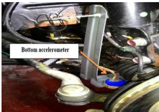
Fig. 4 Accelerometer sensor installation for vertical shaft acceleration
