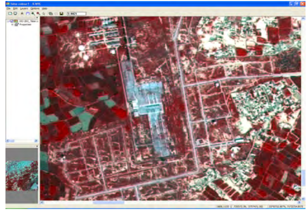
Fig.1 500KV Sheikh Muhammadi Grid Station
