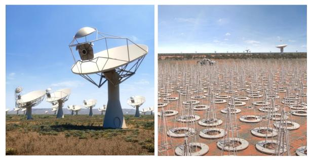
Figure 1. Artist impression of the SKA1 MID antennas in South Africa (left) and SKA1 LOW dipole antenna station in Australia (right).
