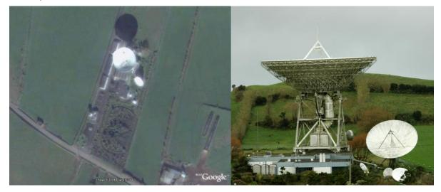
Figure 1. Earth Stations in São Miguel (Azores) – Intelsat Standard A 32-metre parabolic antenna. We can see the waveguide system below the dish.
