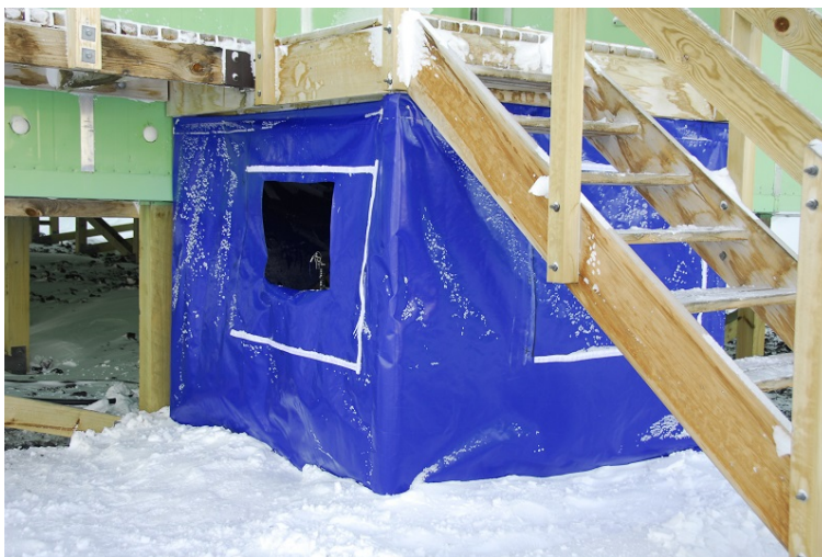
Figure 6.3.: The LP-DOAS telescope was located inside the blue polar tarp, in order to shield it from strong winds and thereby reduce vibrations and jitter, but also to prevent snow from accumulating on top. Photo courtesy of Tim Hay.
