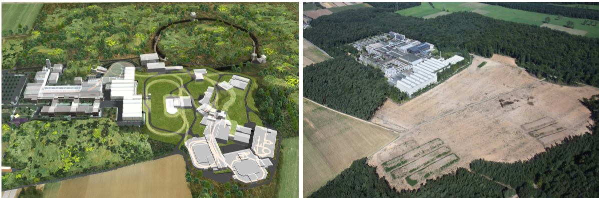
Figure 3.2.: Left: model of the planned FAIR extension together with the already existing GSI facilities. Right: aerial photograph from August 2012, showing the very first stage of construction. Both photos are taken from GSI [3].
