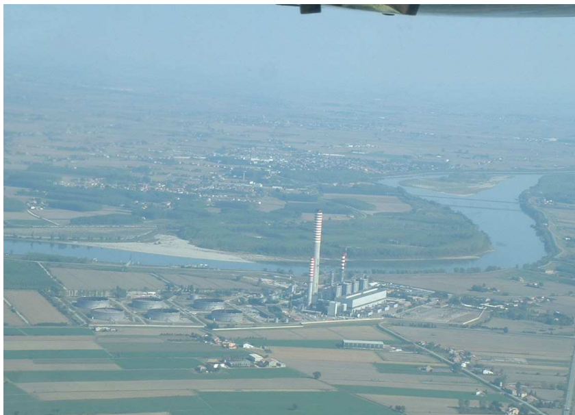
Figure 8-16: Photo of Sermide power plant taken during the second plume flight. As can be seen the visibility is far better than 13 km, which is the distance to the plant during this time. The photo was taken with zooming modus of the camera.
