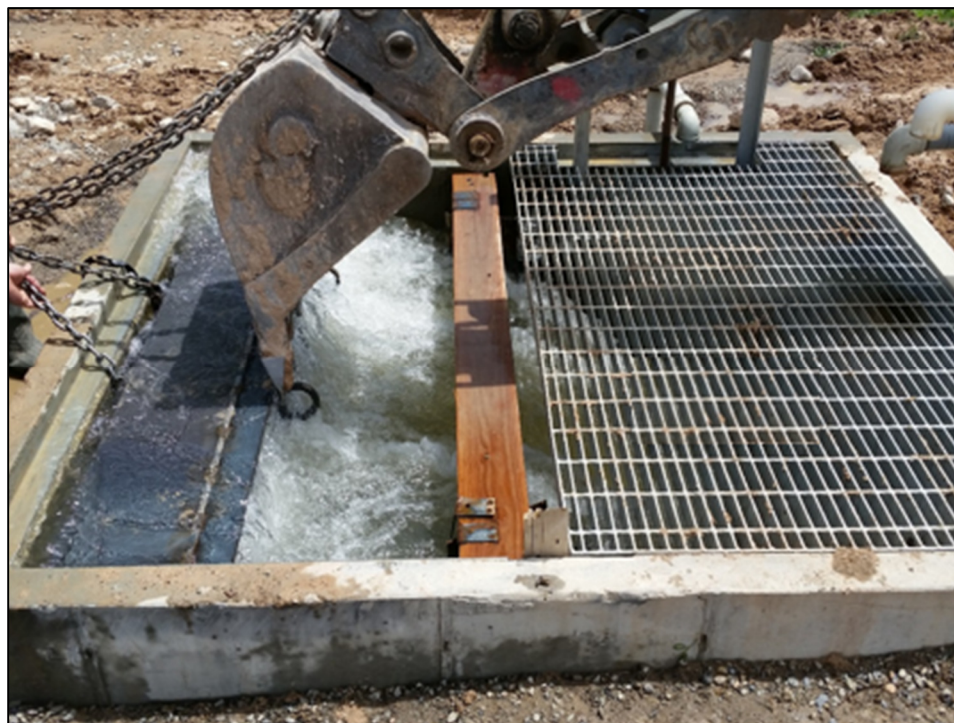
Figure 21. Prototype splitter box after vertical plate was installed.
