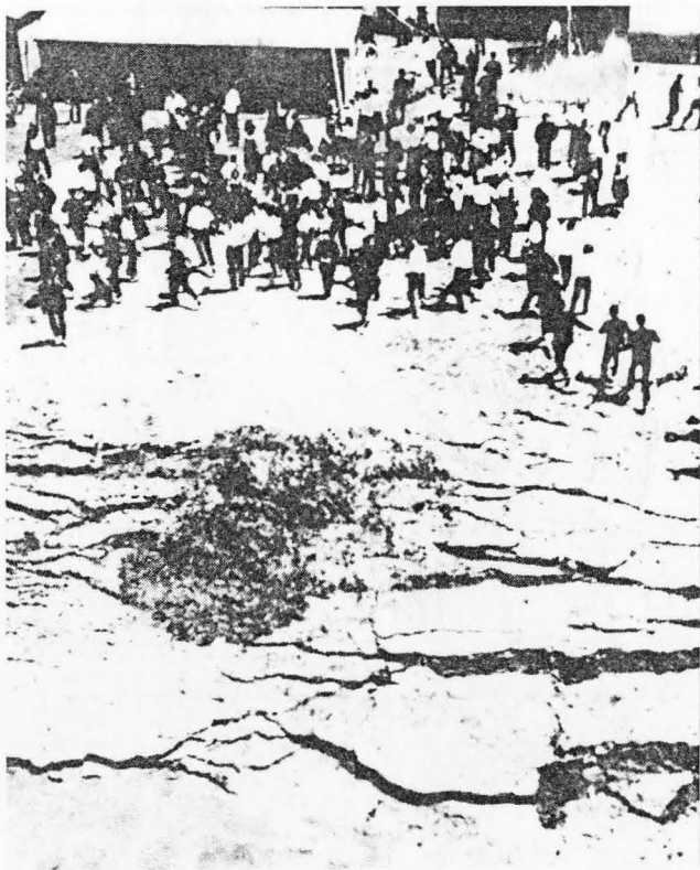
Figure 3. Springs developing during earthquake in Niigata, Japan, 1964 (after Seed and Idriss, 1967).
