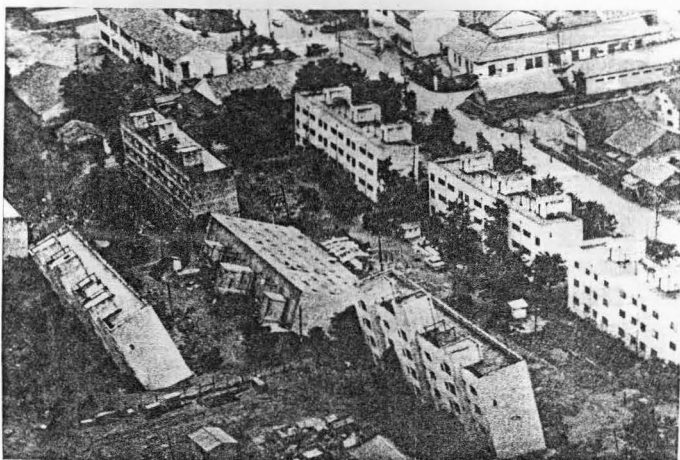
Figure 1. Tilting of apartment buildings in Niigata, Japan, 1964 (after Seed and Idriss, 1967).
