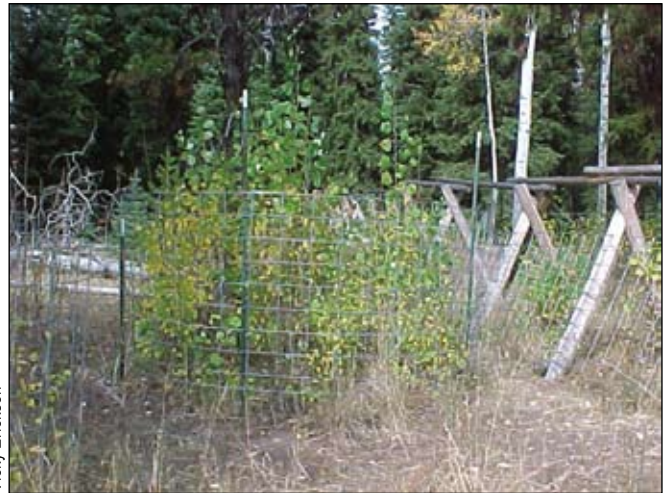
Figure 32—Circular aspen enclosure constructed from two 16-ft welded-wire rod fence panels.
