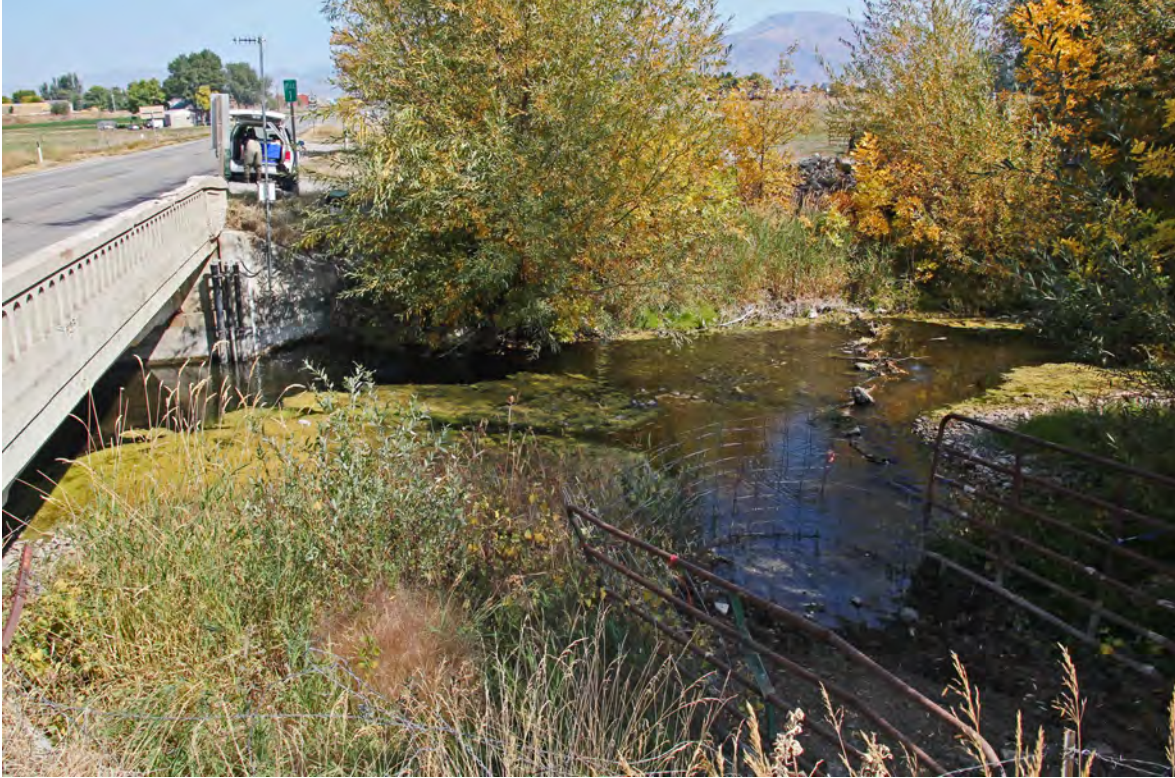
Station 8: Bridge crossing on the eastern edge of Wellsville, Utah
