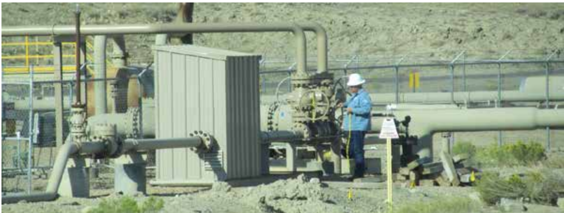
Figure 63: Worker s Servicing Energy Infrastructure near Bonanza, UT. Source: Michael Gottfredson
