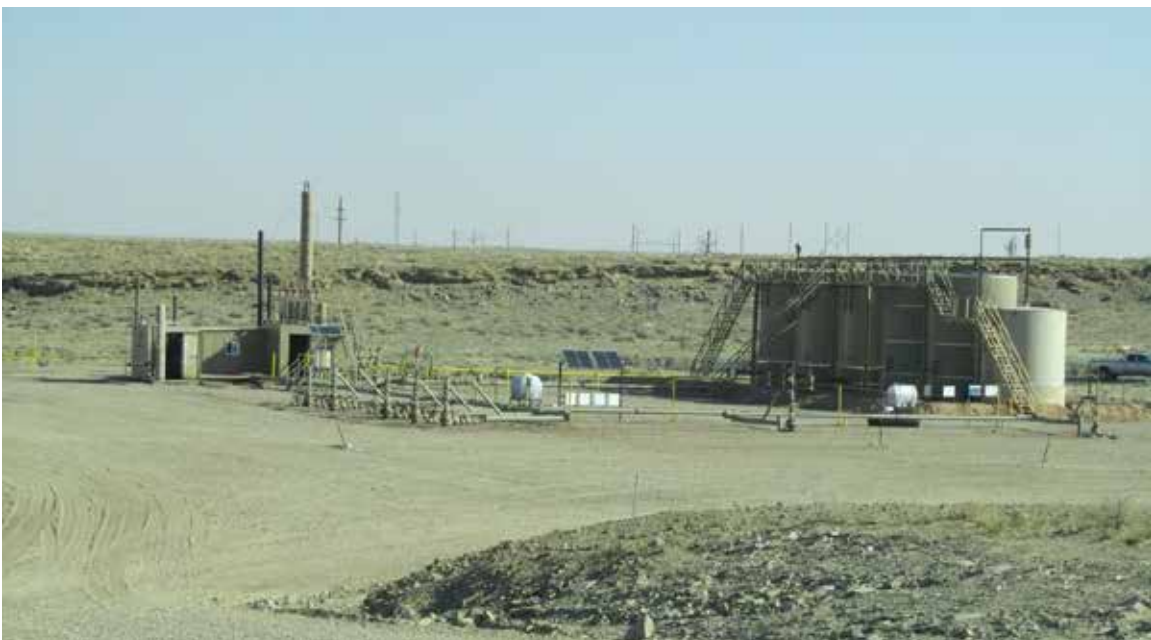
Figure 69: Seven Natural Gas Well Heads on One Pad, Suggesting Directional Drilling, in the Uintah Basin. Source: Michael Gottfredson
