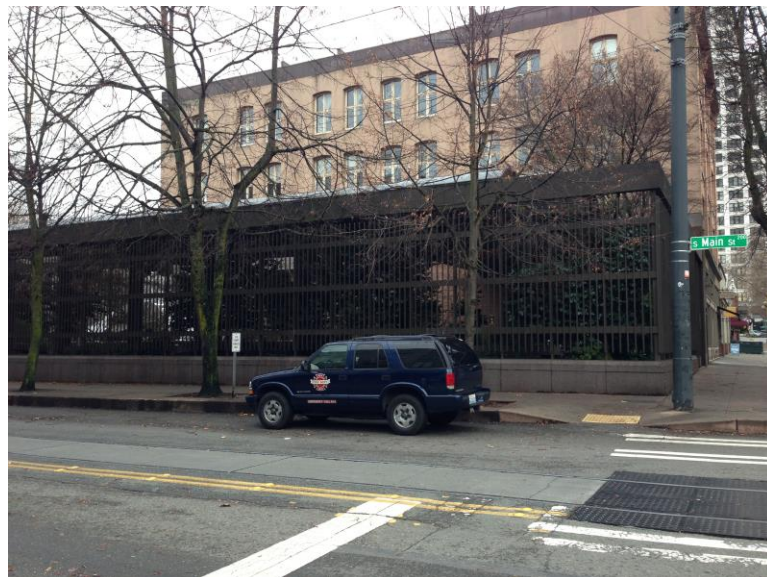
Figure 56. South side. Corner of Waterfall Garden Park. Photo by author.
