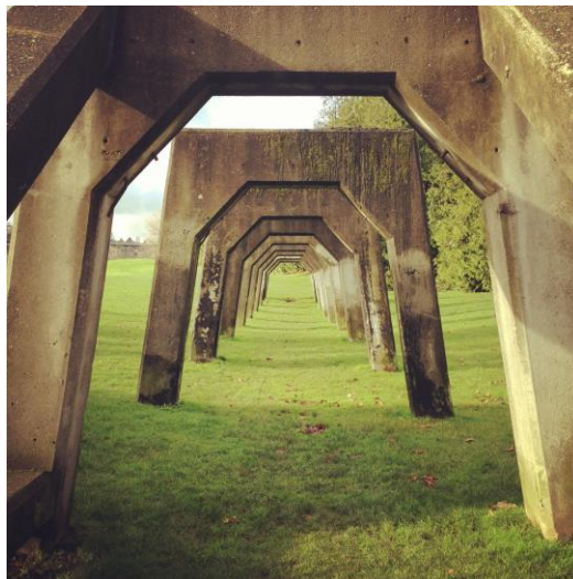
Figure 20. Concrete train trestles. View looking west. Photo by author.
