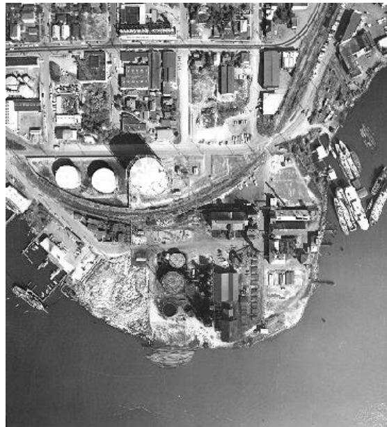
Figure 14. Gasification plant, 1965. Courtesy of Seattle Municipal Archives. Item 2908
