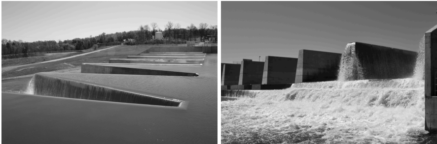
Figure 2 – Staged labyrinth spillway at Lake Townsend, Greensboro, NC, USA
