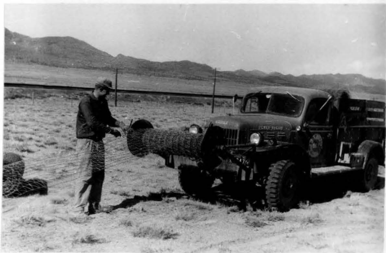
Figure 2. Powered wire roller in operation
