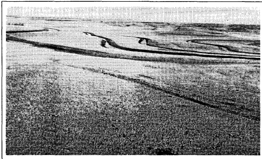
Terraces constructed as part of a RC&D roadside erosion control project reduce runoff, conserve moisture and provide water areas for wildlife.
