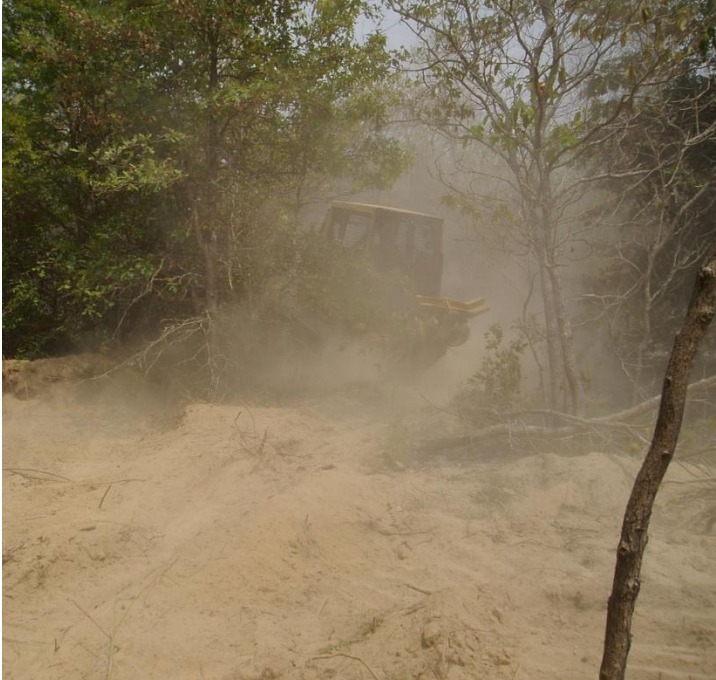
Texas FS Initial Attack 082111 – Particulate exposure during dozer operations
