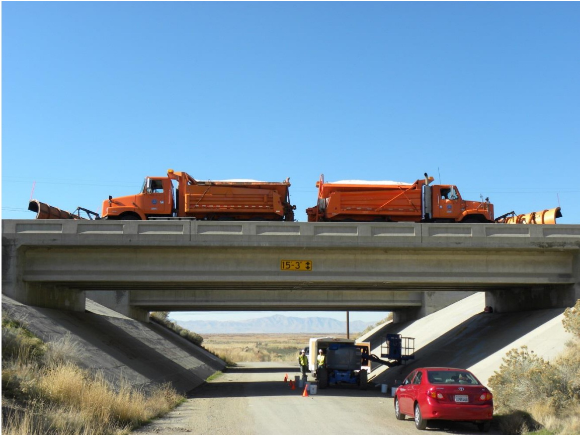
Fig. 1 Utah Pilot Bridge (structure number 1F 205) side view
