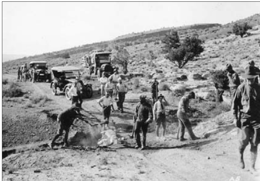
Repairing the road in Tanner's Wash, en route to Lee's Ferry, July 18 or 19, 1923.
