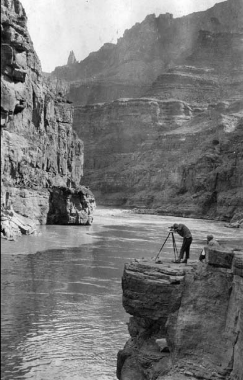
Surveying at 36 Mile Rapid. Burchard is probably the man at the alidade, with Birdseye recording. Freeman snapped this striking image about August 8.
