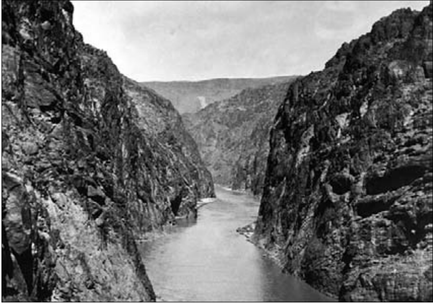
Boulder Canyon Dam site, located in Black Canyon and the present site of Hoover Dam, photographed in 1922 by the U.S. Bureau of Reclamation.
