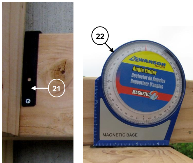
Figure 11. Positioning the magnetic angle-finder (22) onto metal plate 21.
