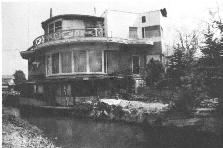
... others completely block access and even hang out over the water.
