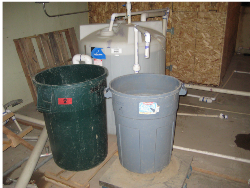
Figure 13. Fill tank on weight scale
