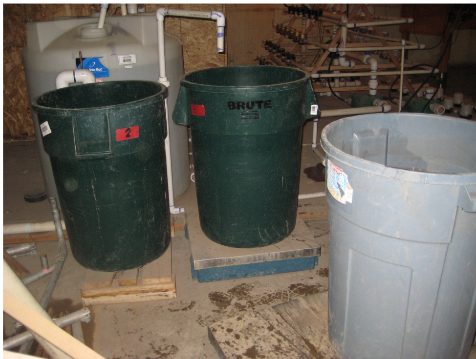
Figure 15. Replace fill tank with empty tank
