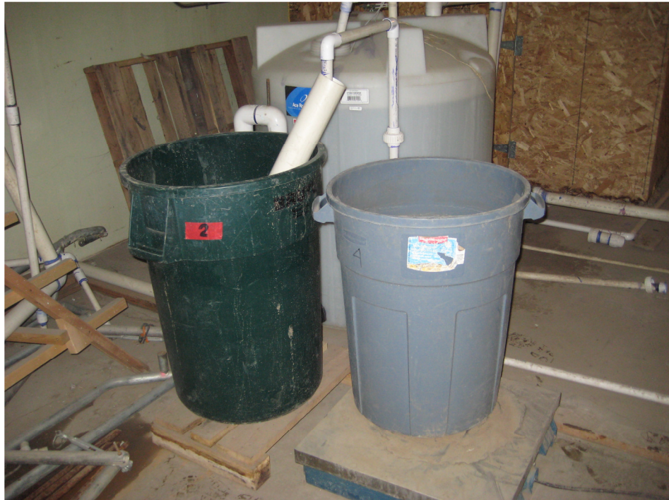
Figure 14. Diverting flow from fill tank
