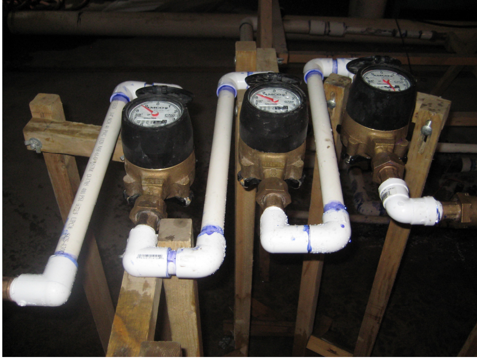
Figure 7. Two 90 degree elbows in plane
