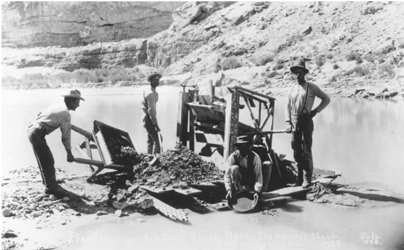
From the simple gold pan to the rocker and improvised wheelbarrow, technology became increasingly important as men worked the land to yield its riches. This staged photo at “Dempsey’s claim” in July 1894 illustrates the equipment used in the earlier years of gold mining on the river. (Charles Goodman photo, Manuscripts Division, Marriott Library, University of Utah)
