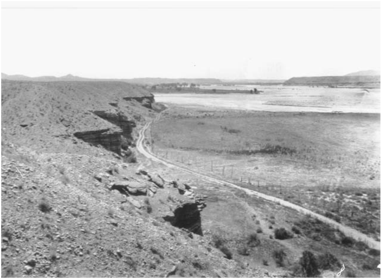
This 1928 photo shows part of the abandoned Colorado-Utah road one mile below the mouth of McElmo Creek, looking upstream towards Aneth. Notice both the scarcity of vegetation along the river and the road's susceptibility to flooding. (Herbert E. Gregory photo, #558, U. S. Geological Survey)
