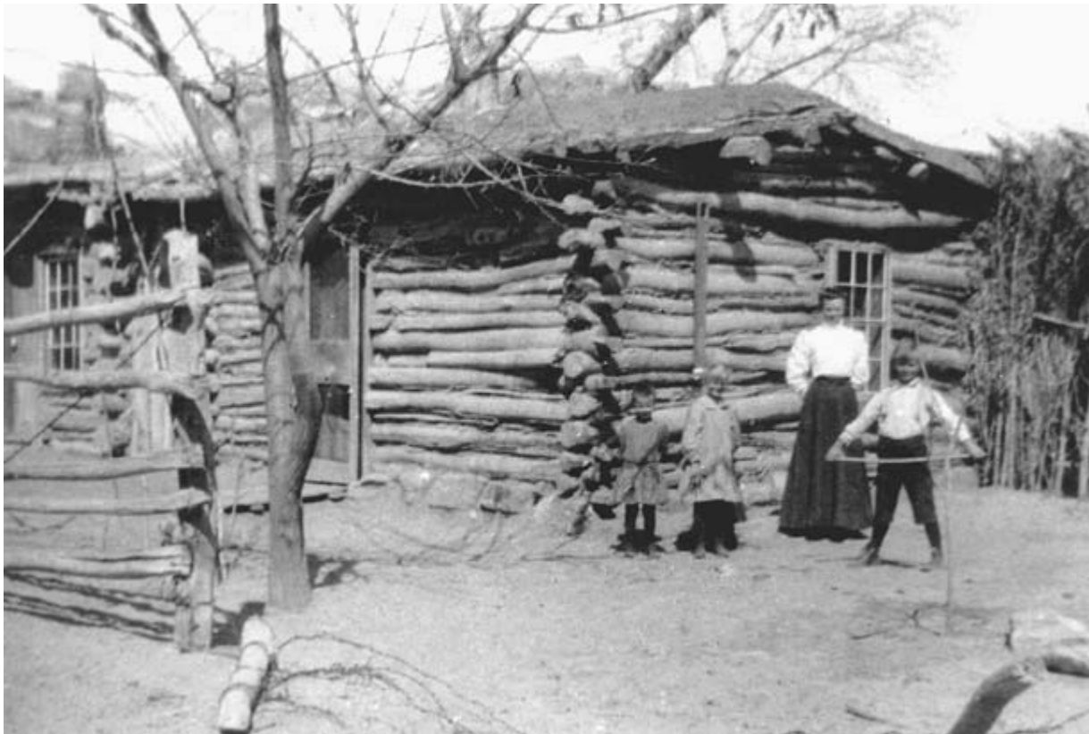
The early home of the Wayne H. Redd family in Bluff illustrates building with what Albert R. Lyman called “that rams-horn breed of trees . . . whose walls bowed in and out with wonderful irregularity.” (San Juan Historical Commission)
