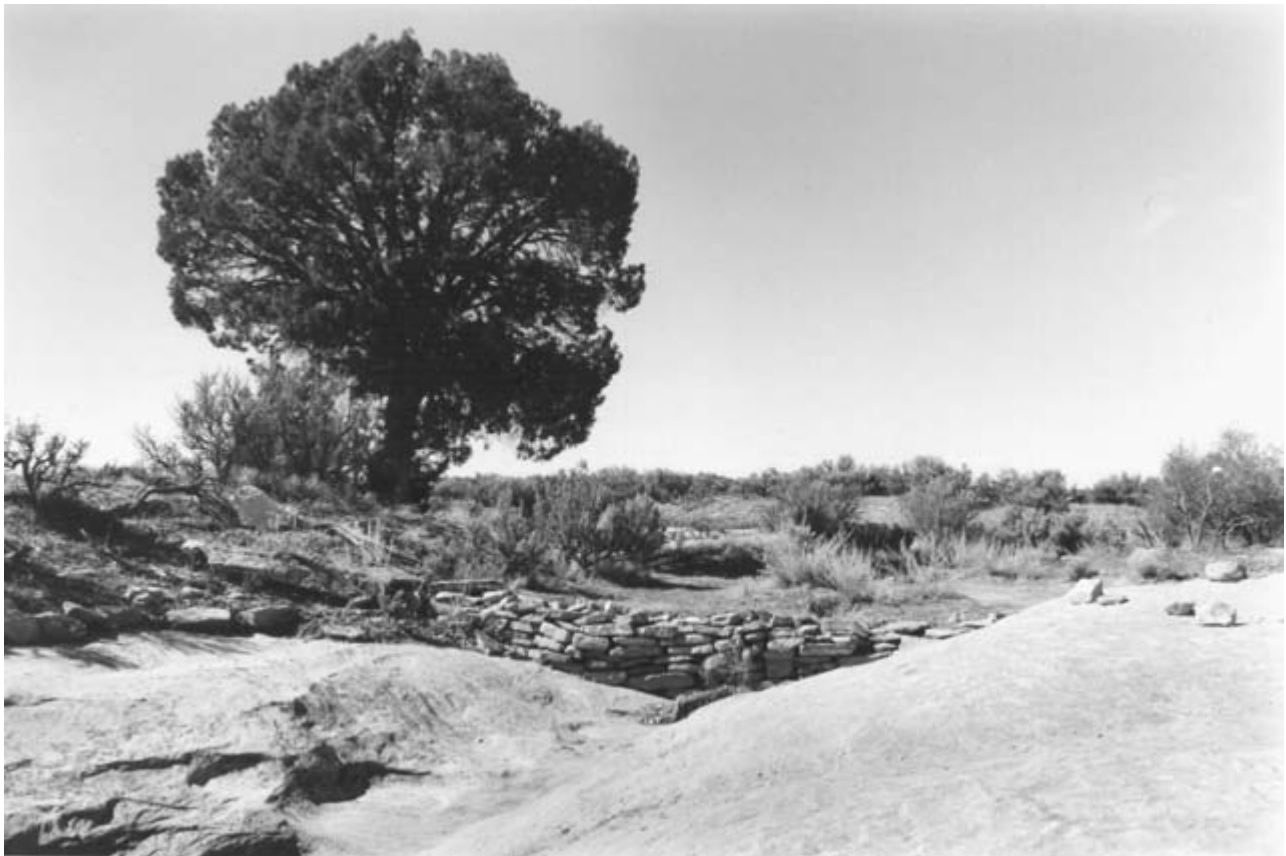
The Anasazi used check dams like this reconstructed one at Hovenweep (facing page) to catch precious water in an arid environment. (James M. Aton photo)
