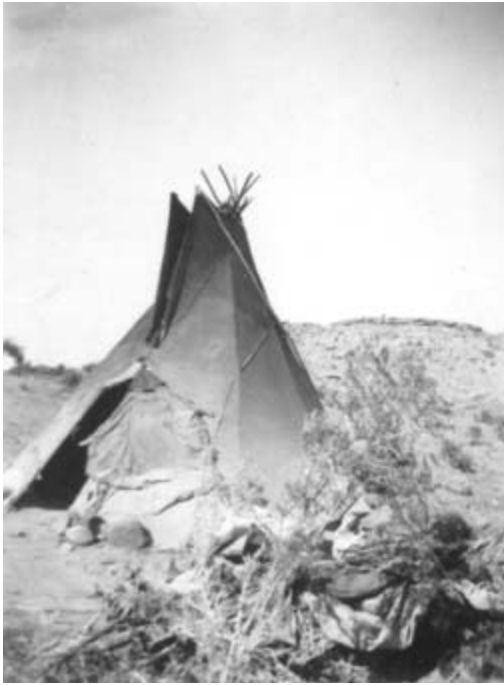
Southern Ute tepees, made of deer and elk skins, served as winter quarters for the people as they sought lower elevations and protection from winter storms. (San Juan Historical Commission)
