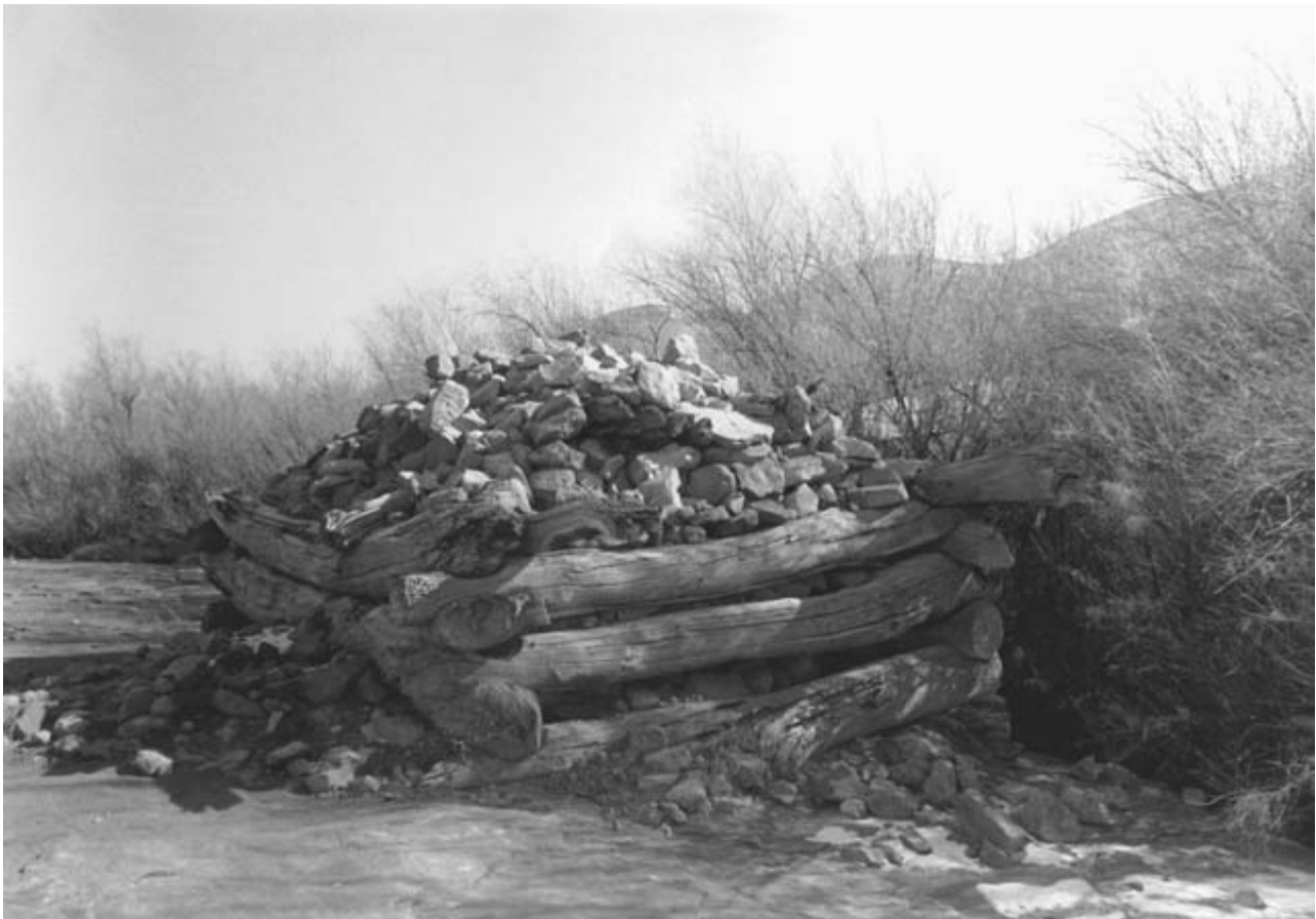
All that is left of the waterwheel system at the Hyde-Barton Trading Post, where the San Juan passes through Comb Ridge, is this anchor of logs and rocks. Many of the posts supplied some of their subsistence by cultivating crops. (James M. Aton photo)
