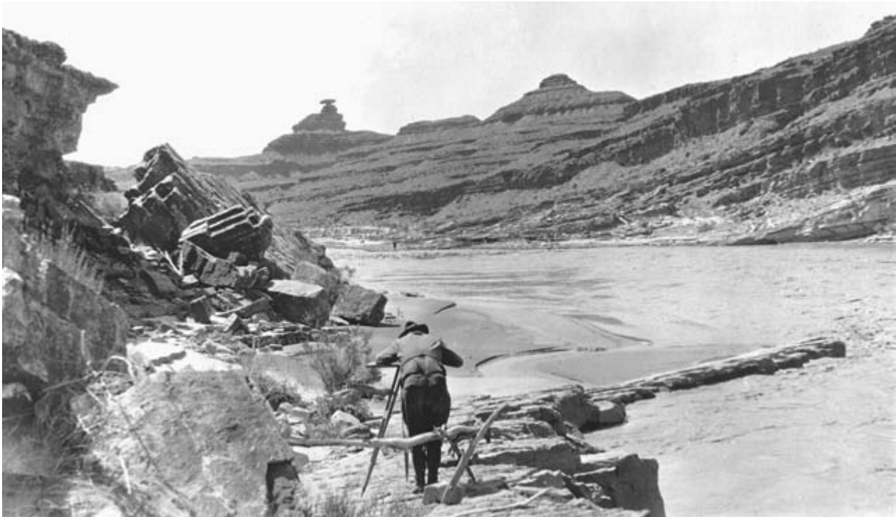
Hugh D. Miser of the 1921 Trimble Expedition works a plane table below Mexican Hat Rock. Note the rod-man across the river. Miser wrote the classic text for the expedition and was the acknowledged “glue” of the trip. (Robert Allen photo, #570, U.S. Geological Survey)
