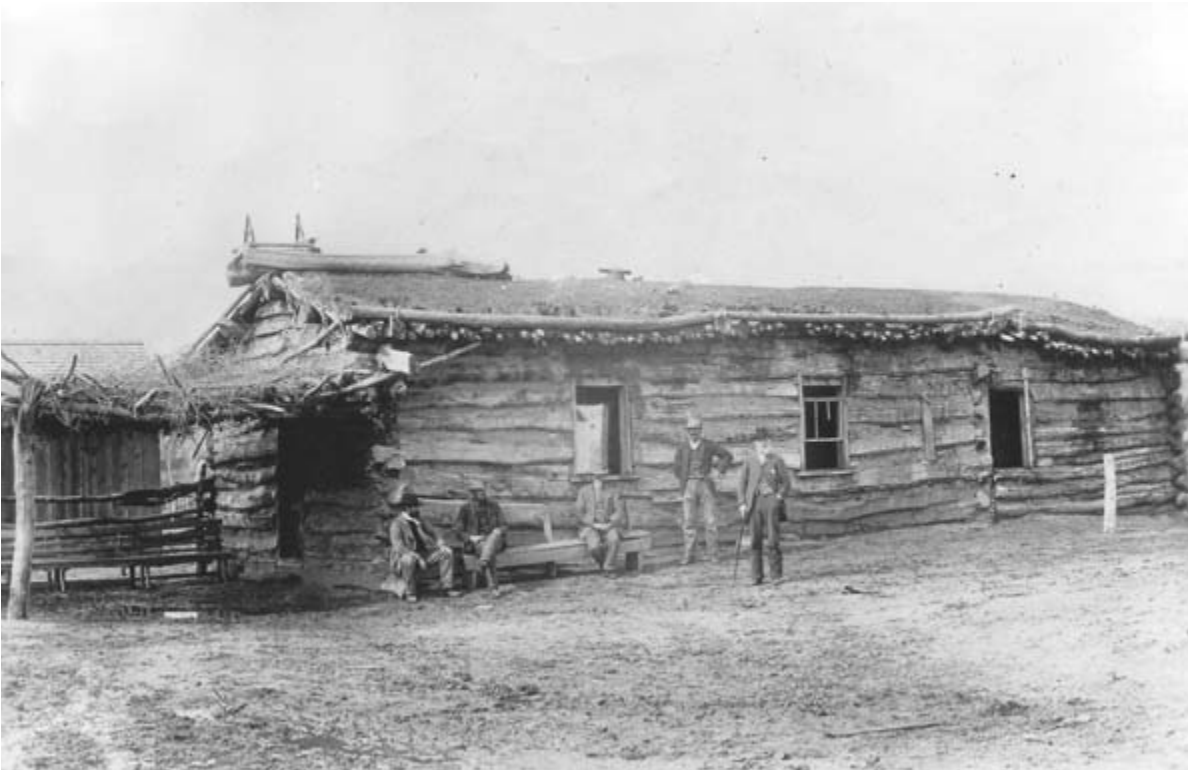
Built in the fall of 1880, this structure for fourteen years served the pioneers as a church, school, dance hall, and public meeting place. Old veterans of the Hole-in-the-Rock ordeal and settlement of Bluff are pictured (left to right): Kumen Jones, Platte D. Lyman, Jens Nielson, James B. Decker, and Francis Hammond. (Charles Goodman photo, San Juan Historical Commission)
